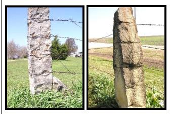
The limestone known as <u>post rock</u> has had many uses other than for the construction of fence posts. The material's durability makes it an excellent building material.
